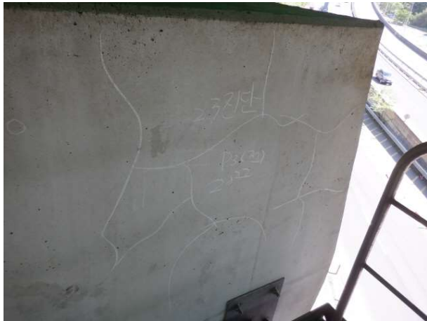
P3 코평 망상균열( A=1.0 \times 1.0=1.00\text{m}^2 )
