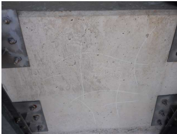
P2 코평 망상균열( A=0.8 \times 0.8=0.64\text{m}^2 )
