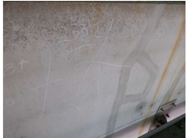
P3 코평 망상균열( A=0.5 \times 0.5=0.25\text{m}^2 )
